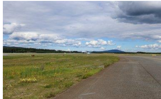
Degradation of de-icing chemicals on the side areas.
