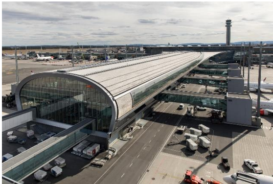
Great need for charging options at apron.
