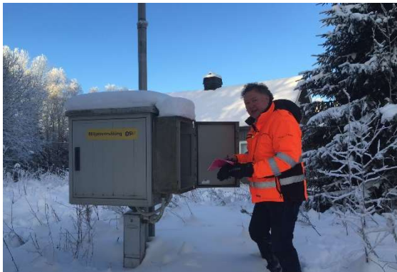
Oslo Airport's NTMS records the aircraft noise level continuously at 11 points around the airport
